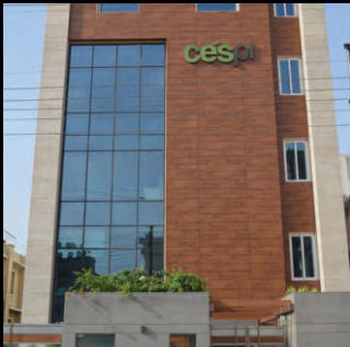
CESPL Building (LEED certified Building) Noida, Uttar Pradesh
