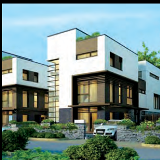
Villa Bilaspur, Chhattisgarh
